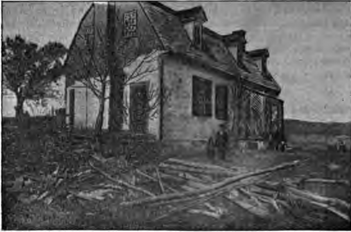
OLD HOUSE AT BROAD CREEK, MD. 200 years old.
